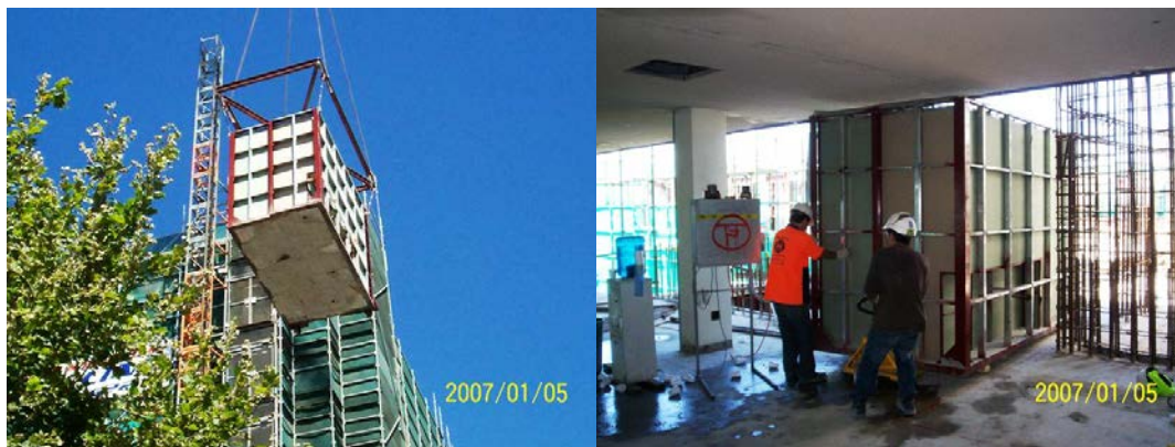
Figure 21 - Arrival of the first Module (Source: John Smolders)
