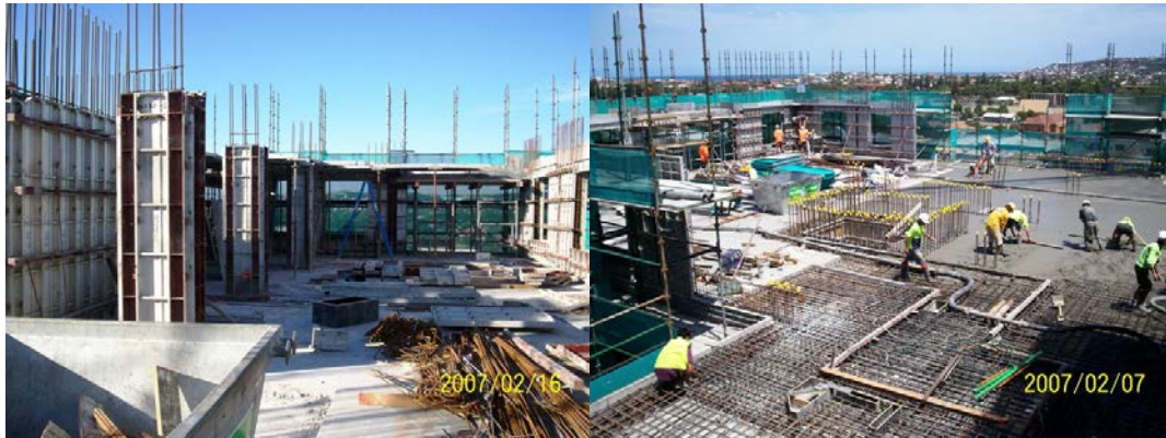
Figure 24 - Aluminium Formwork system-pictures (Source: John Smolders)
