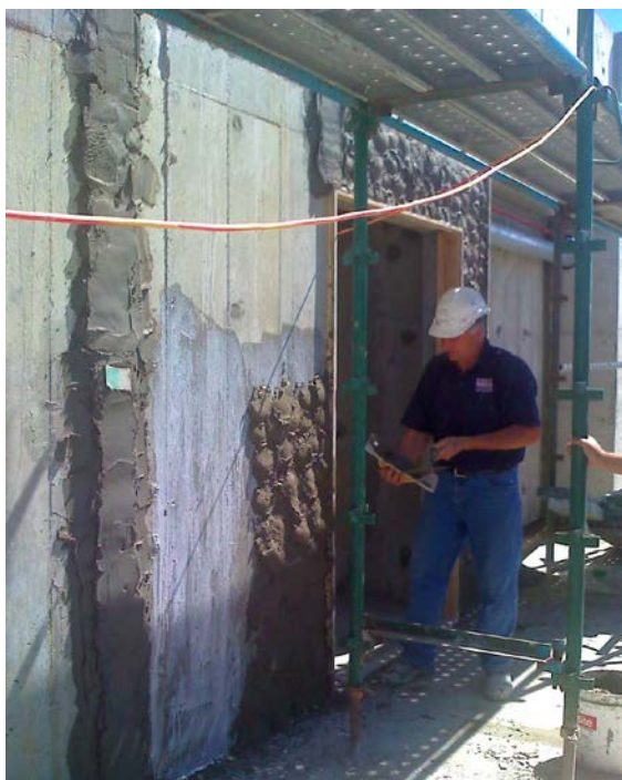
Figure 25-Realigning Wall to be Vertical (Source: John Smolders)
